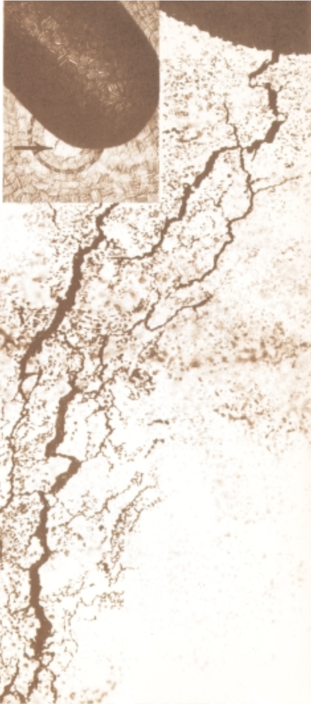
Stress corrosion cracks at the bottom of a tube cavity in an aluminum rotor
