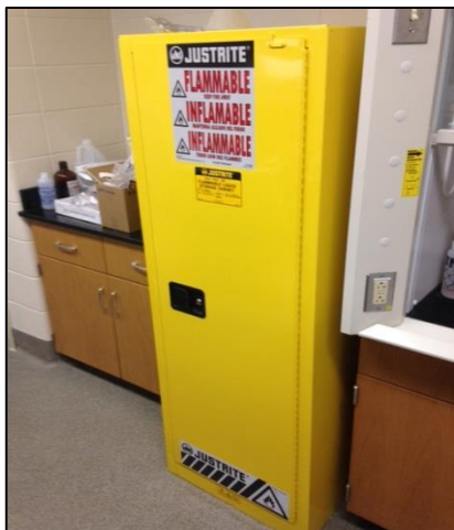
Figure 5.1 – Flammable Storage Cabinet
