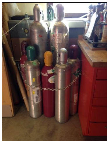
Figure 5.3 – Not In-Use Cylinders
