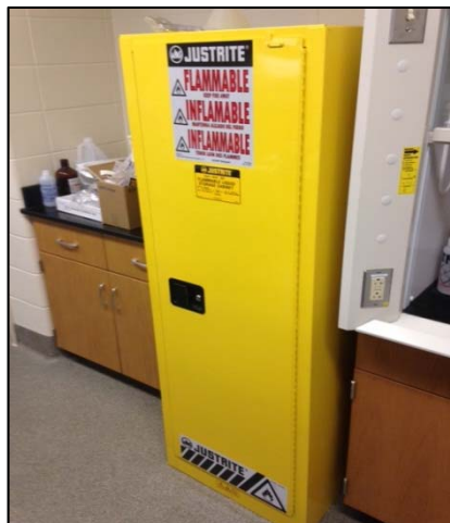
Figure 5.1 – Flammable Storage Cabinet
